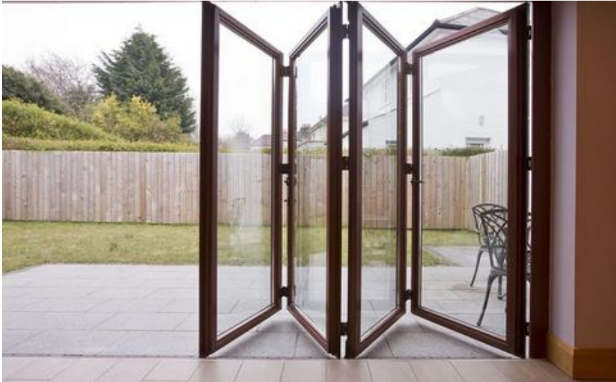
Figure 17 Collapsible doors
