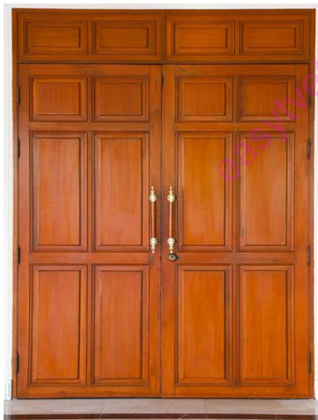
Figure 6 Framed and paneled door
