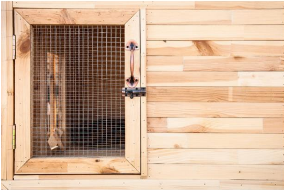
Figure 9 Wire gauzed door
