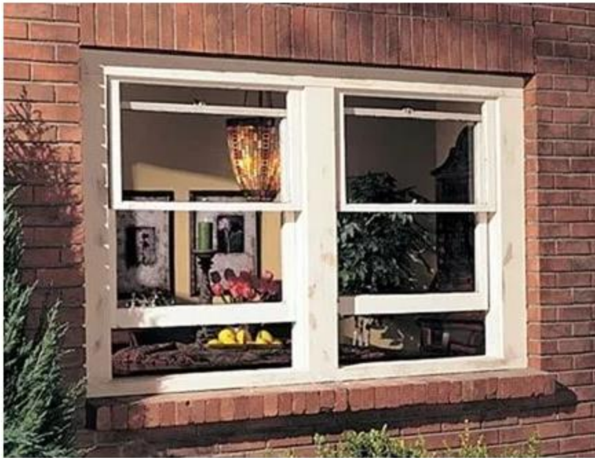
Figure 24 Double Hung Windows
