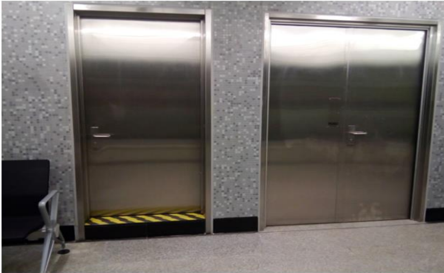
Figure 14 Steel plate door
