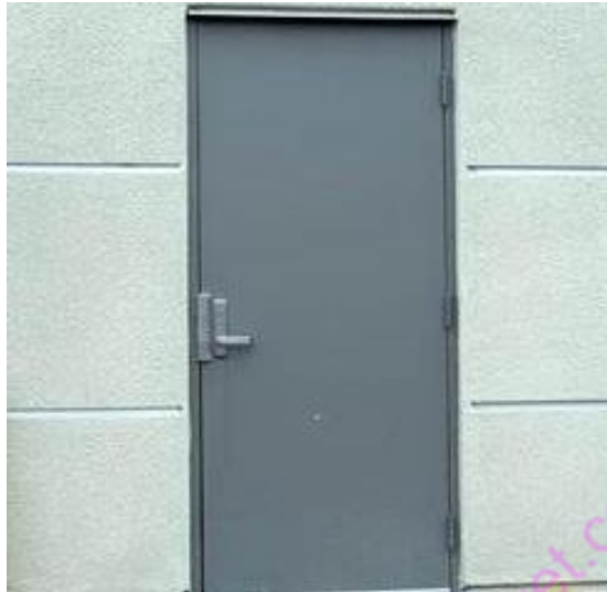
Figure 13 Hollow metal door
