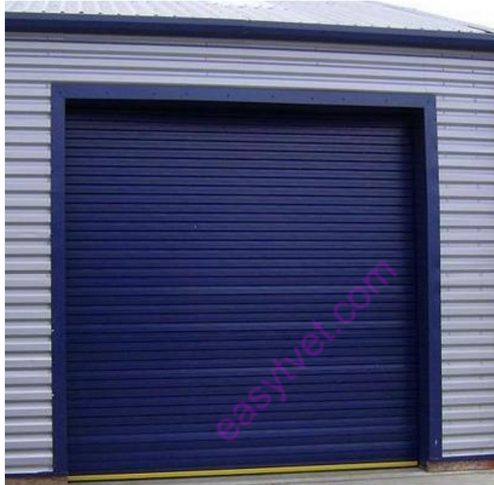
Figure 16 Rolling shutters
