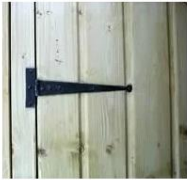
Figure 49 Garnet Hinge
