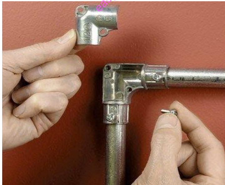
Figure 38: Additional Step to Install a Pulling Elbow
