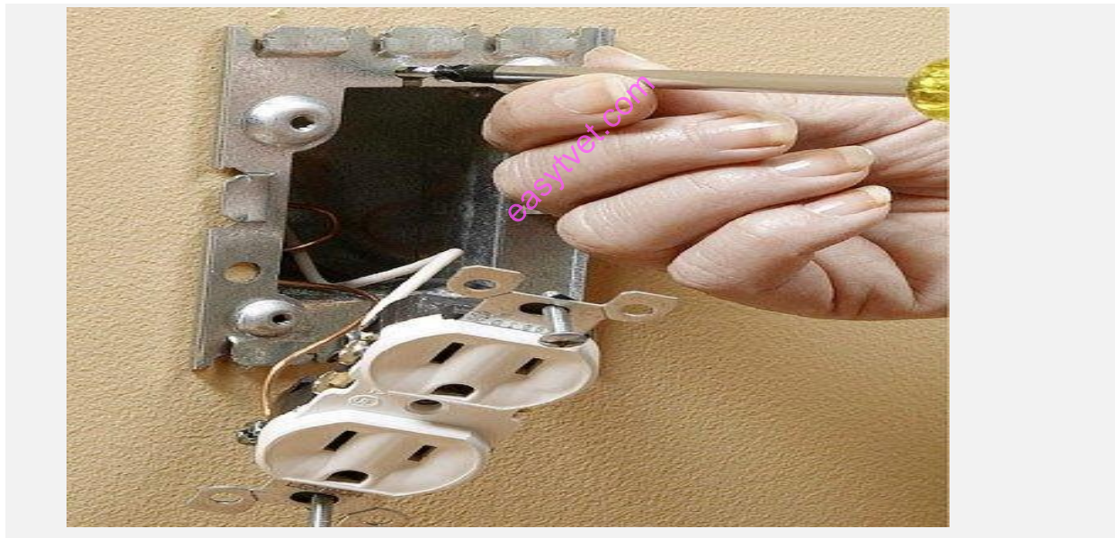
Figure 46: Step, Install Raceway Starter Box
