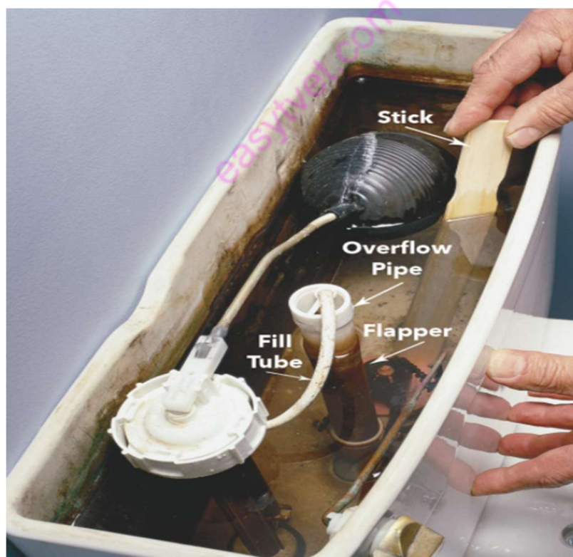
Test the flapper
